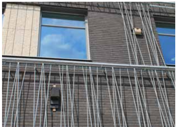
△ The new office block contributes to local biodiversity through its green roofs and walls.
