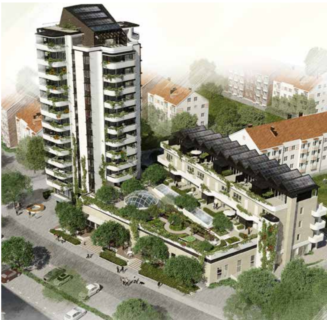
△ Greenhouse, a part of Ekostaden Augustenborg in Malmö, comprises a 14-storey tower block, 12 terrace housing units and a pre-existing building converted into new social facilities. The roof is fitted with 200 m 2 solar cells.
